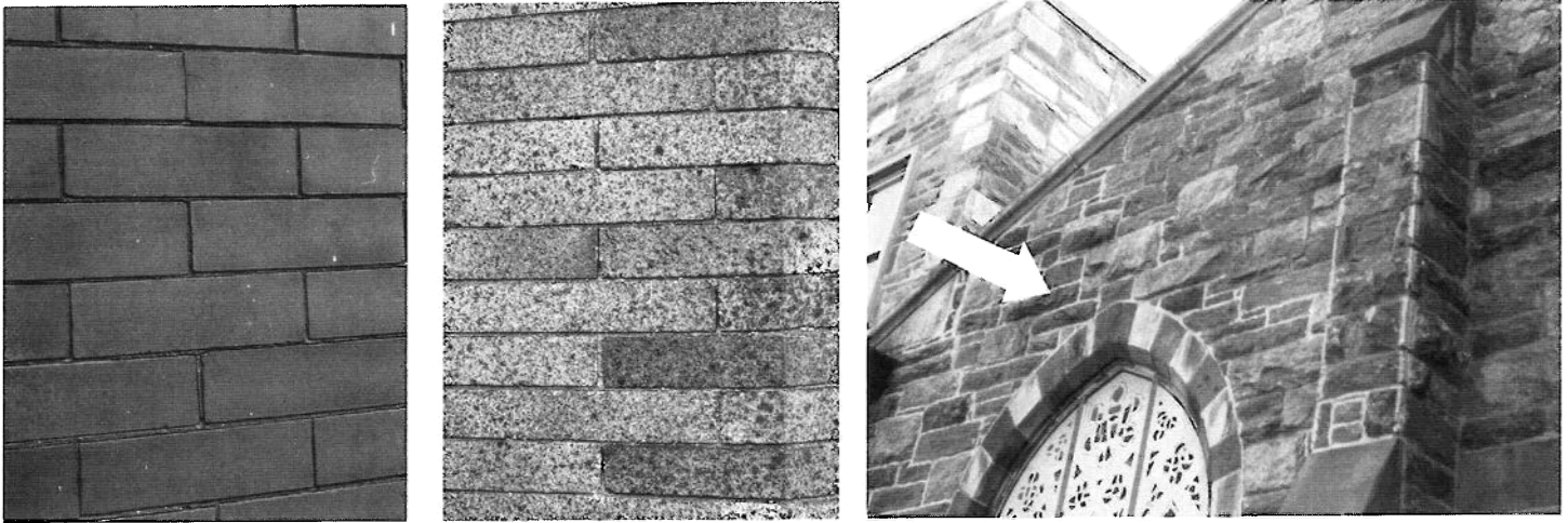
Figure 6. Tinted mortar. (left) Black mortar with a beaded joint was used here on this late-19th century hard pressed red brick and, (center) a dark brown tinted mortar with an almost flush joint was used on this early-20th century Roman brick. (right) When constructed at the turn-of-the-century, this building was pointed with a dark gray mortar to blend with the color of the stone, but the light-colored mortar used in spot repointing has destroyed this harmony and adversely impacts the building's historic character. Photos: Anne Grimmer.
