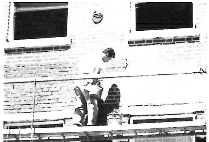
Figure 17. This photograph shows the significant visual change to the character of this historic brick building that has resulted from improper repointing procedures and a noticeably increased thickness of the mortar joints. Photo: Lee H. Nelson, FAIA.
