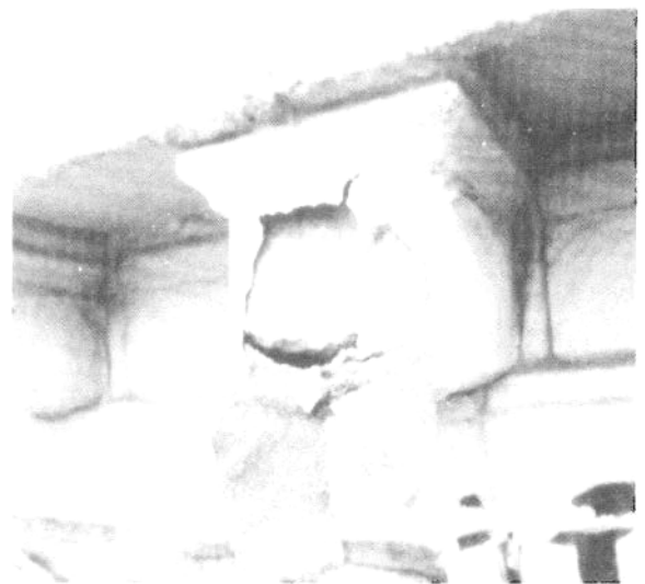
Figure 27. Instead of correcting the roof drainage problems, an elastomeric coating was applied to the already saturated limestone cornice. An elastomeric coating holds moisture in the masonry because it does not "breathe" and does not allow liquid moisture to escape. If the water pressure builds up sufficiently it can cause the coating to break and pop off as shown in this example, often pulling pieces of the masonry with it. Photo: National Park Service Files.
