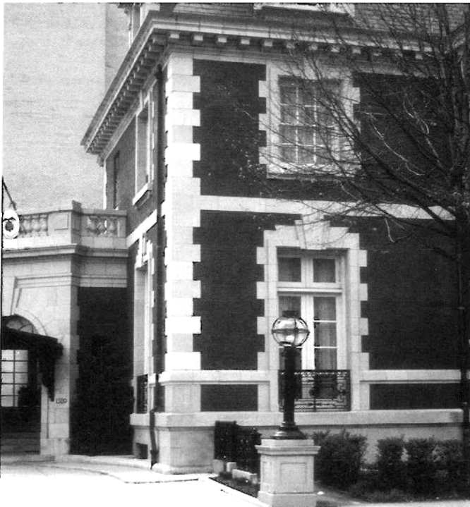
Figure 4. The foundation of this brick building is limestone, but the decorative trim above is architectural terra cotta intended to simulate stone.
