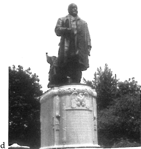
Figure 16. (a) The limestone base was heavily stained by runoff from the bronze statue above. (b) A poultice consisting of copper stain remover and ammonia mixed with fuller's earth was applied to the stone base and covered with plastic sheeting to keep it from drying out too quickly. (c) As the poultice dried, it pulled the stain out of the stone. (d) The poultice residue was removed carefully from the stone surface with wooden scrapers and the stone was rinsed with water. Photos. John Dugger.
