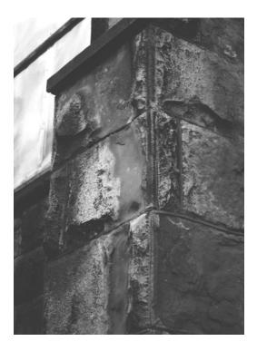
■ Unchecked water drainage will result in rapid deterioration of sandstone and brick.
