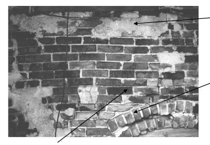
Careless application of mortar obscures the bond pattern of the brick
