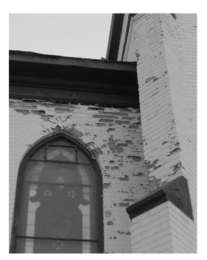
■ Here brick has been severely damaged by inappropriate sandblasting and painting (see MA 5, MA 3).
